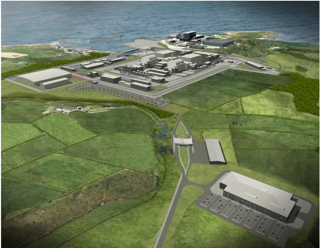
Figure 0-4 Aerial impression of the Power Station
